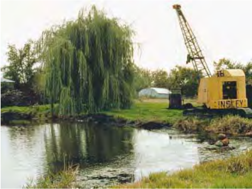
A dragline equipped with a clam bucket can deepen shoreline areas around ponds. Be sure to remove dredge spoils from the area to prevent them from washing back into the water.
