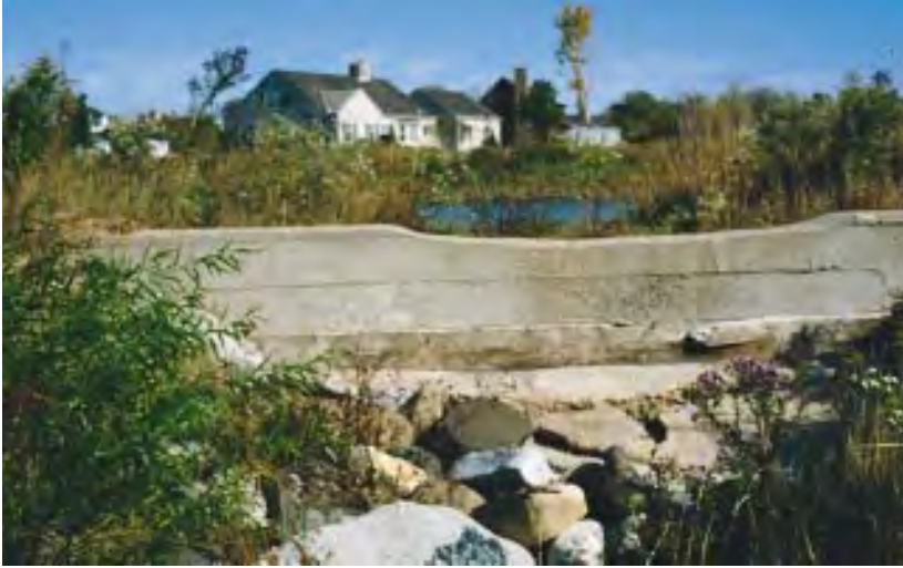
A cement spillway carries away excess water.
