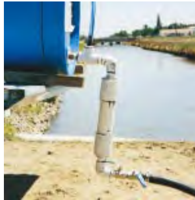
A simple drip system attached directly to a drum of Cutrine-Plus.
