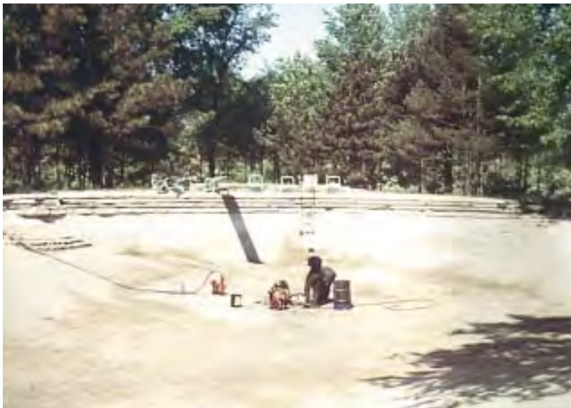
Sealing a pond with Bentonite clay.
